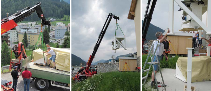
Figure 7.1: Impressions from the installation of the heliostat structure
